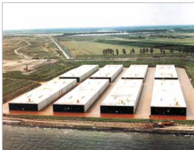
Fot. 7. Gotowe elementy tunelu Liefkenshoek (Hydronic)
