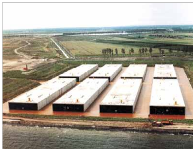
Fot. 7. Gotowe elementy tunelu Liefkenshoek (Hydronamic)
