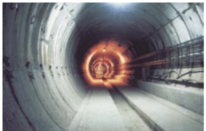
Fig. 3. Metro tunnel with reinforced concrete tubing
