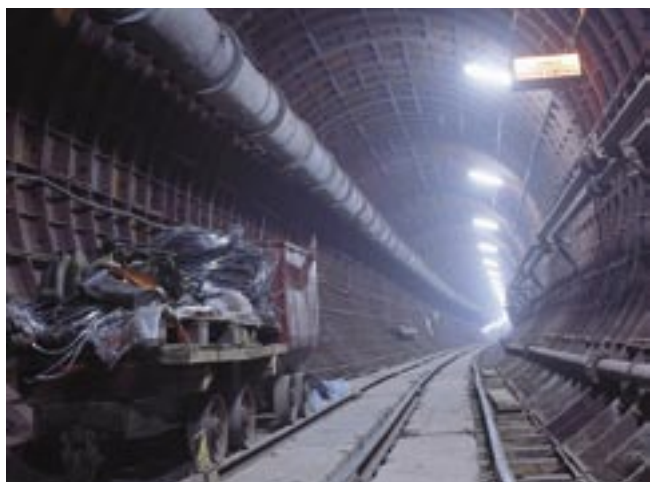
Fig. 7. Tunnel under construction
