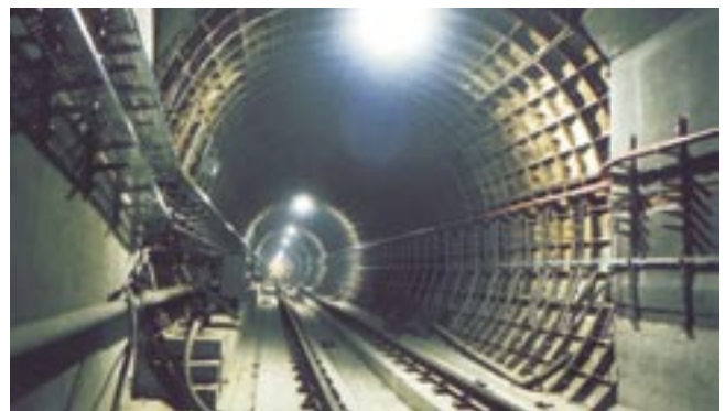
Fig. 2. Metro tunnel with cast-iron tubing
