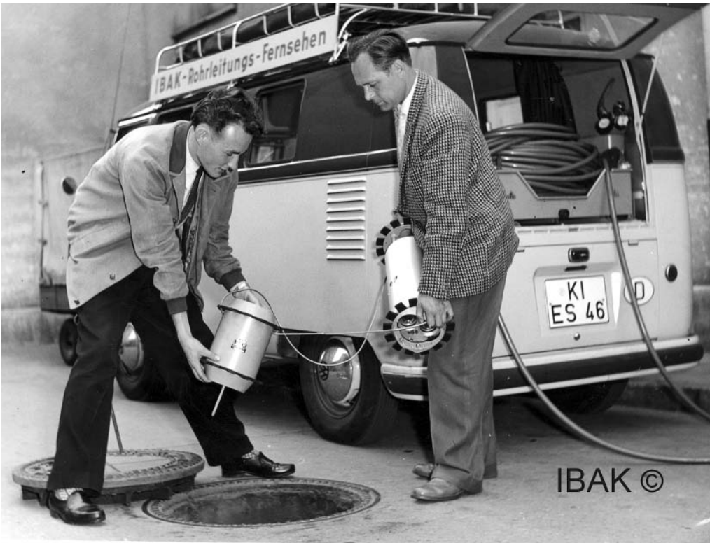
Photo 1. First sewer inspection camera + additional lightning world-wide
